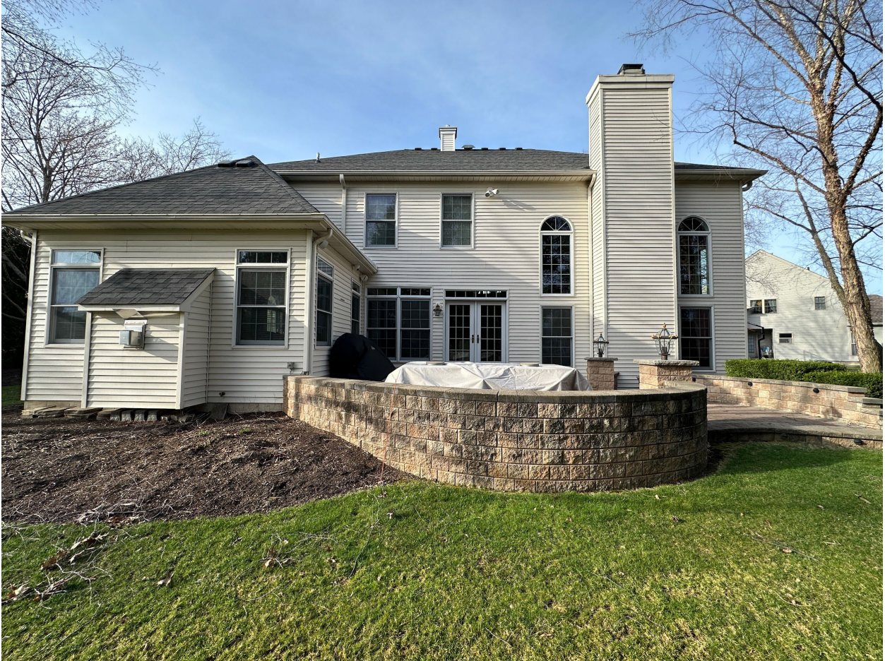
REAR VIEW OF 31729 MARITIME COURT. PROPOSED PORCH WILL EXTEND 2' FROM EXISTING PATIO WALL LOCATION
