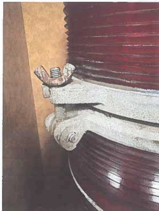
open for bulb replacement
