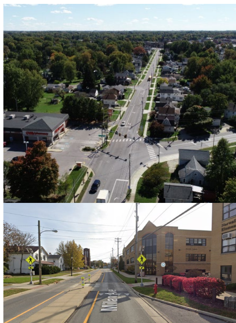
RRFB midblock pedestrian crossing
