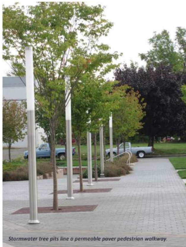
Stormwater tree pits line a permeable paver pedestrian walkway. Photo Credit: EPA Green Stormwater Solutions for Congregations
