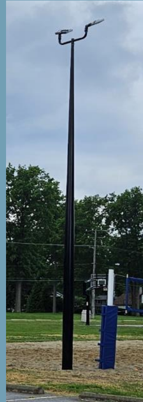
Northern Parking Lot Lighting • 1 Poles In Center; 3 shorter
